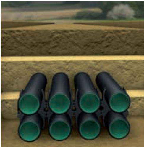
Kabuflex conduits are installed underground in a gravel-sand mixture, and covered with a layer of mechanically compacted soil.
